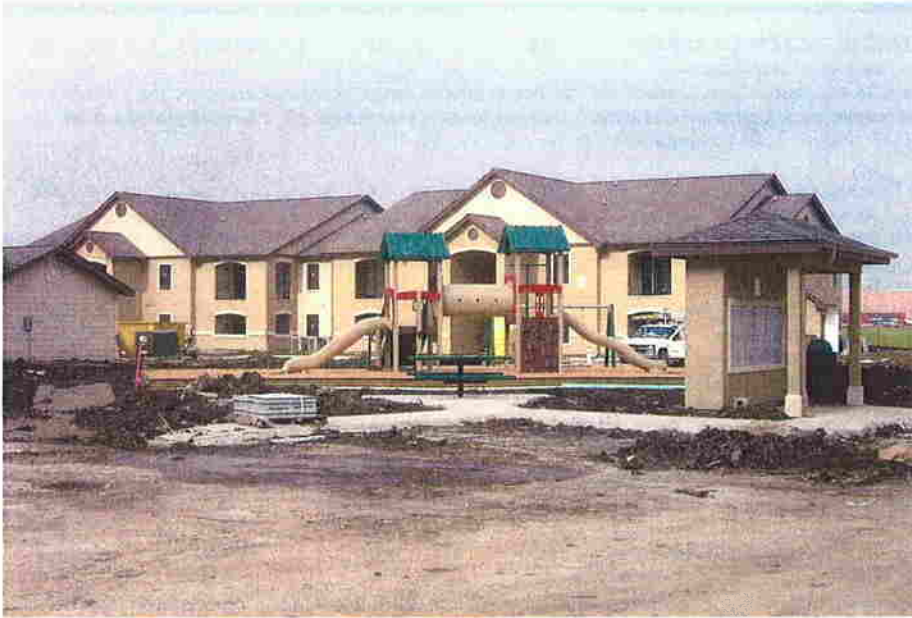
Realtex Development Corp.'s Sunset Way Apartments, the first project to break ground in the Gulf Opportunity Zone, is set to open May 1 in Port Arthur, Texas.
